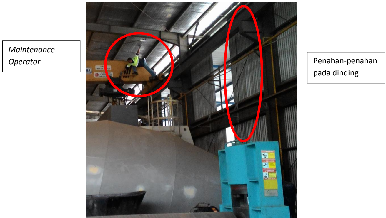
Gambar 5.1 Maintenance Operator Saat Memperbaiki Overhead Crane
