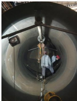
Figure 2.12 Setting Cone Assembly
