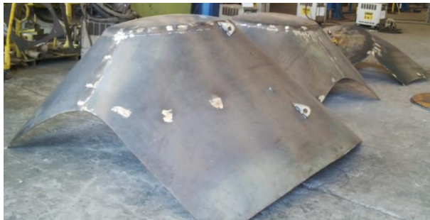
Figure 2.10 Welding The Cone With Bottom Flanging
