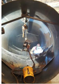
Figure 2.14 Full Weld Assembled Cone
