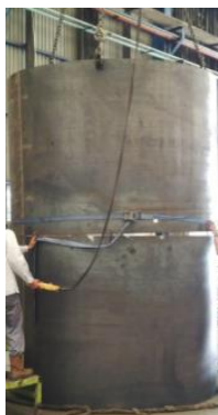
Figure 2.7 Welding Material to Make a Tank
