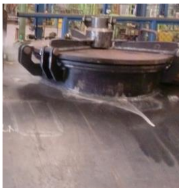
Figure 2.16 Full Weld Man Hole
