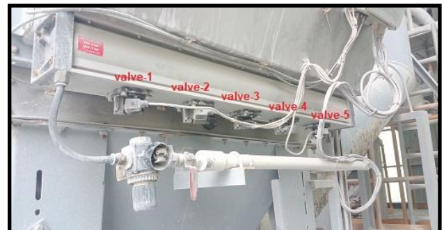
Gambar 8. Posisi Solenoid valve
